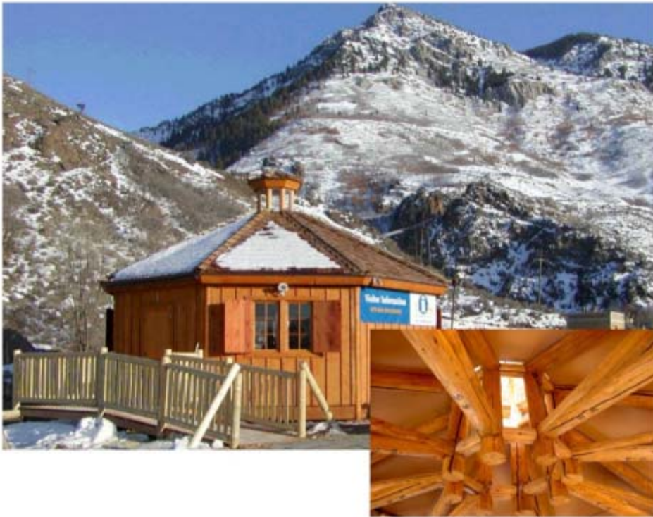
Figure 2. Several demonstration structures using small-diameter roundwood trusses have been built in the United States. This visitor information center in the Wasatch Mountains near Ogden, Utah uses an innovative cupola design (see insert) that ties the roundwood rafters together through the use a ring-like structure below the cupola. Photo courtesy of the U.S. Forest Products Laboratory
