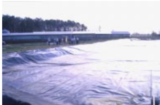
Methane-recovery systems can generate energy from biogas.
