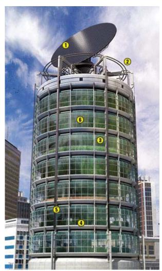
Troughs collect runoff for filtration.
